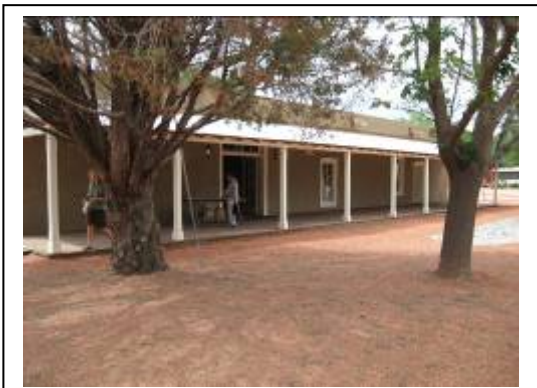
Hubbell House after the renovations
